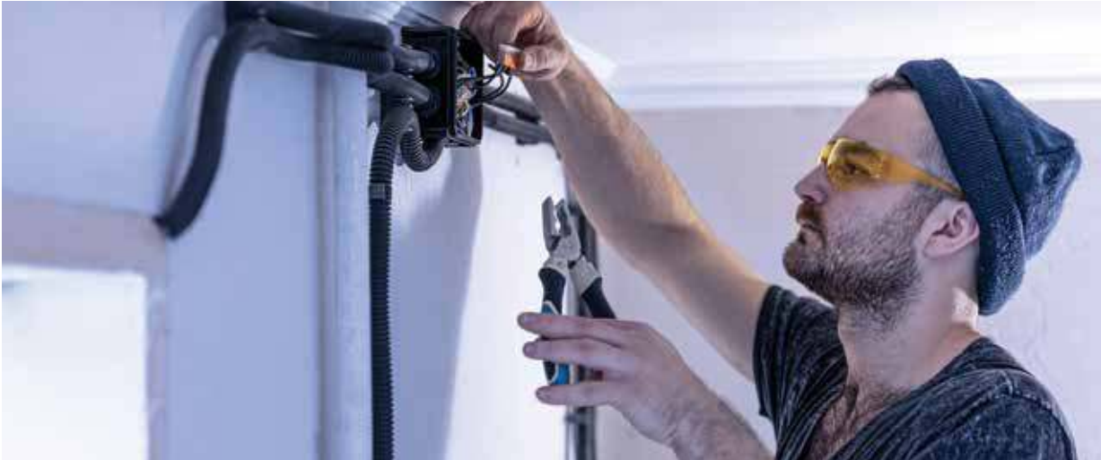
Critical maintenance and repair work during COVID-19.
